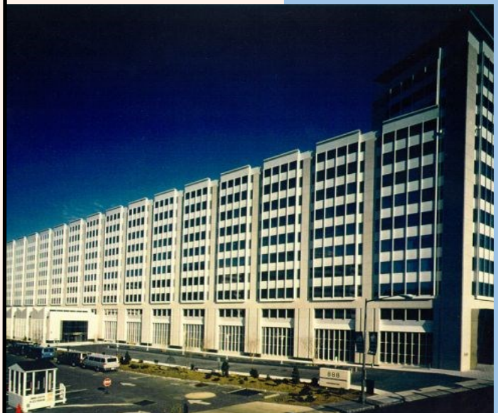
Federal Energy Regulatory Commission Bldg, Washington, DC
